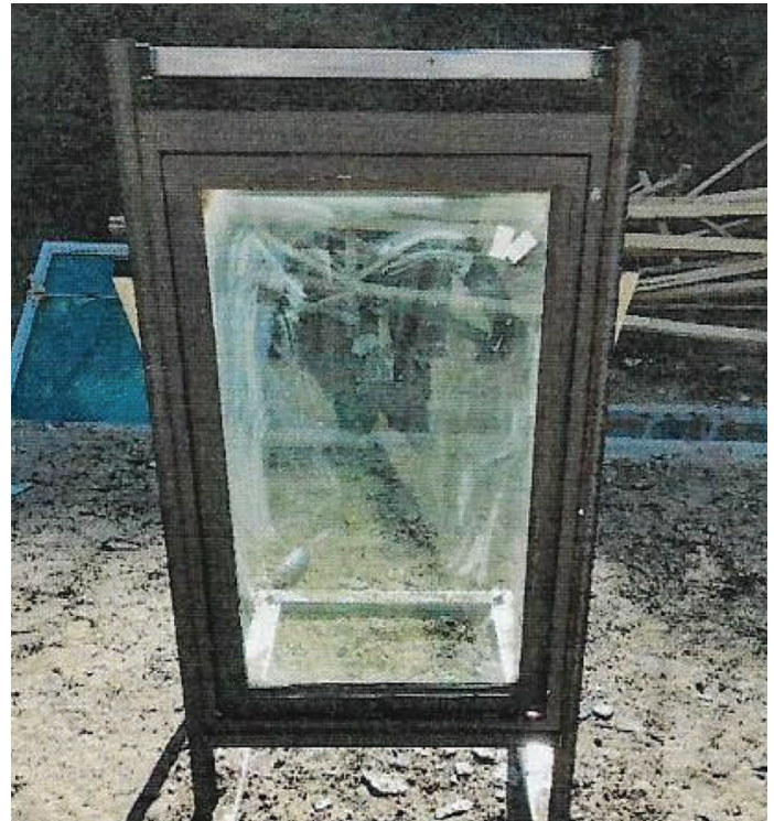
Image 2: Aluminum alloy blast-resistant window after explosion test
