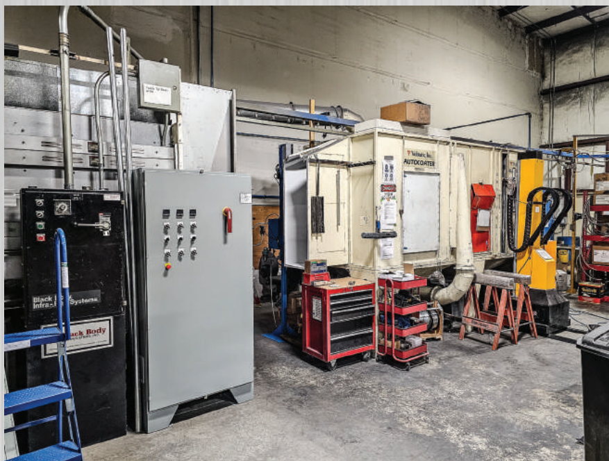
IN-HOUSE POWDER COATING
